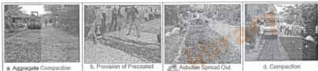
Figure 8. The Sequence of Main Job for Butur Seal
